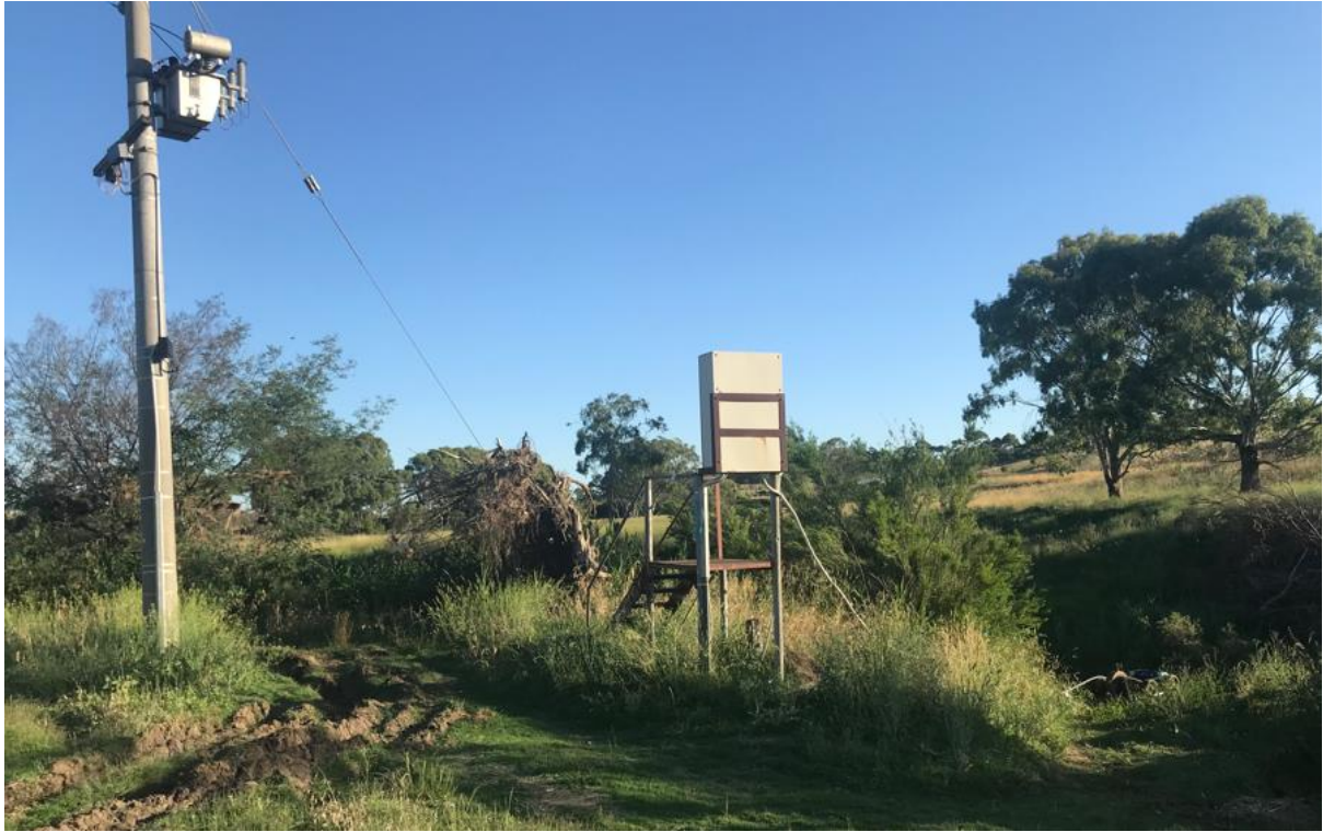
Mains power pole, switchboard, pump installation at far right, debris evident on power pole strain wire
