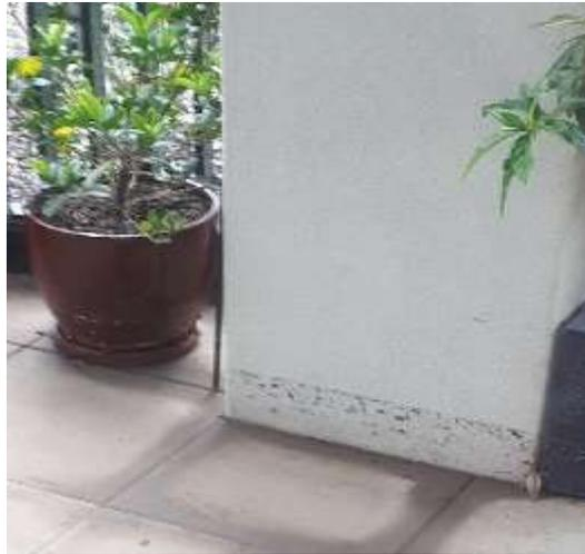
Rear courtyard in Blueridge, post flood. Black sludge left by 6" water from backyard drain pit.
