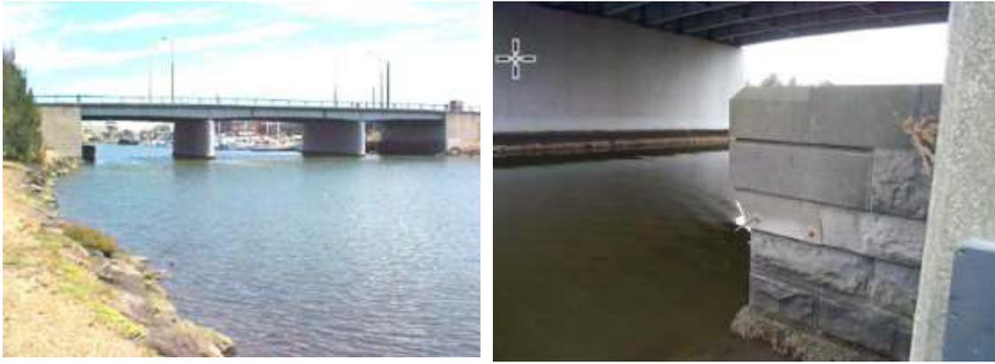
Figure 50: Location of hydraulic improvements to Footscray Road, including downstream end of bluestone abutment to be removed.
