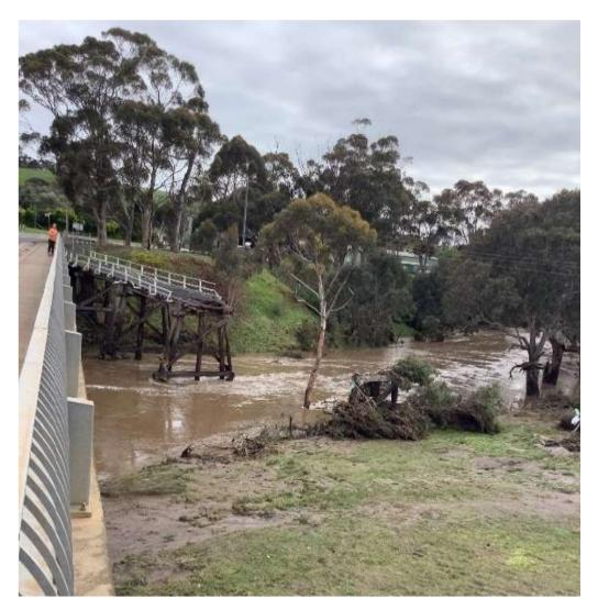
Figure 7: Photo of destruction of Arundel Heritage Bridge post Flood Event. (Source: Submission #60).
