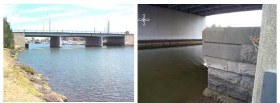
Figure 50: Location of hydraulic improvements to Footscray Road, including downstream end of bluestone abutment to be removed. (Source: GHD 2003 report supplied by VRC).
