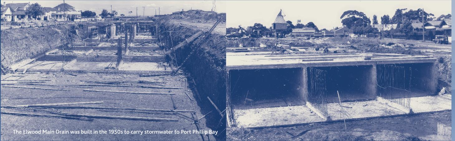
The Elwood Main Drain was built in the 1950s to carry stormwater to Port Phillip Bay
