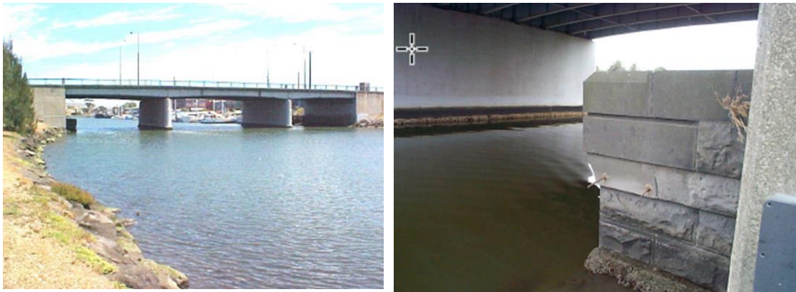
Figure 4: Location of hydraulic improvements to Footscray Road, including downstream end of bluestone abutment to be removed.
