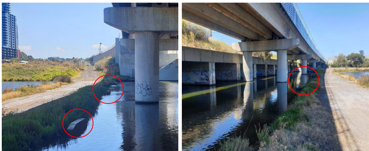
Figure 3-3: Downstream of the Footscray Rail culverts: facing west (left) and east (right). Balancing culverts under the access track circled in red (photos taken in 2023).
